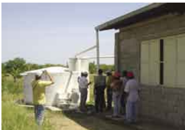
Figure 6: Rainwater cistern with some essential characteristics
