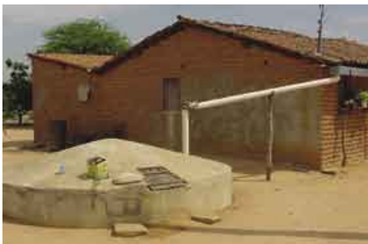
Figure 5: Rainwater cistern with one eave connected to catchment area despite roof with two slopes
